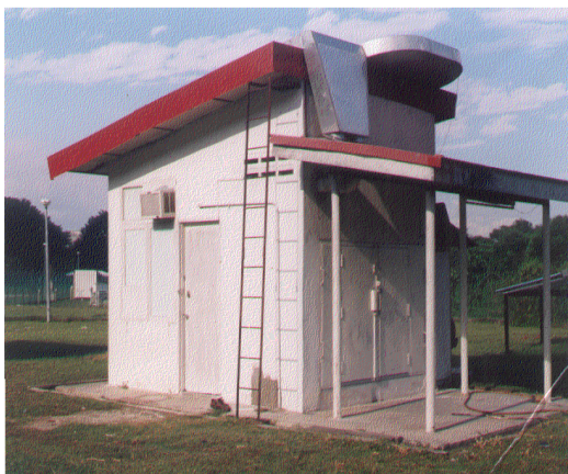
Fig.1: Photograph the solar assisted drying system.
